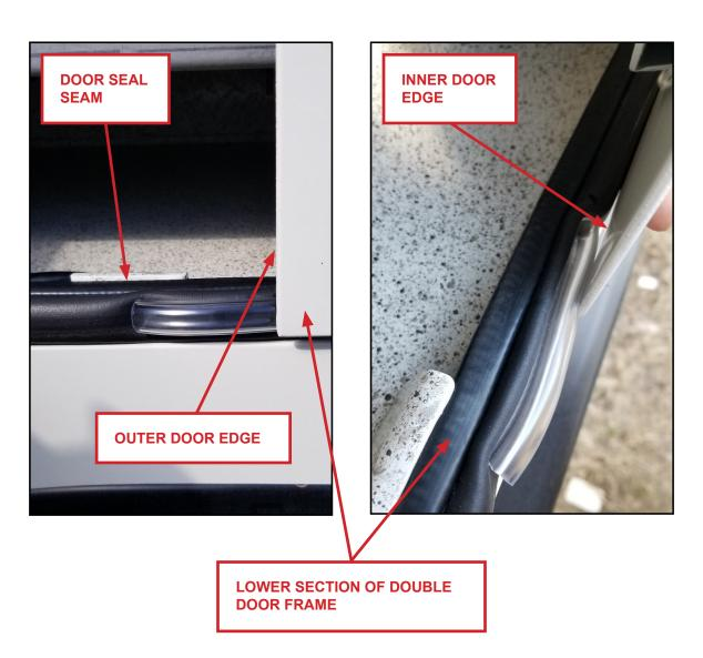
How to install vinyl tubing and silicone the seams:
