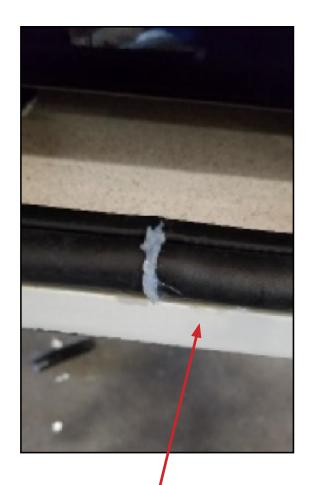
WHEN THE TWO SEAMS ARE PUSHED TOGETHER, INSTALL BOTH SEAM ONTO THE DOOR FRAME EDGE TRIM.
