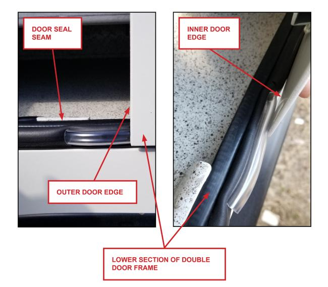
How to install vinyl tubing and silicone the seams:
